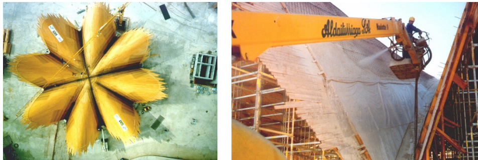
Figure 5: Left: Formwork and partially placed reinforcement. Right: Shotcreting
