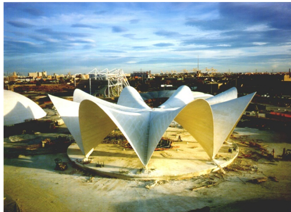
Figure 4: The finished shell prior to building the cladding.
